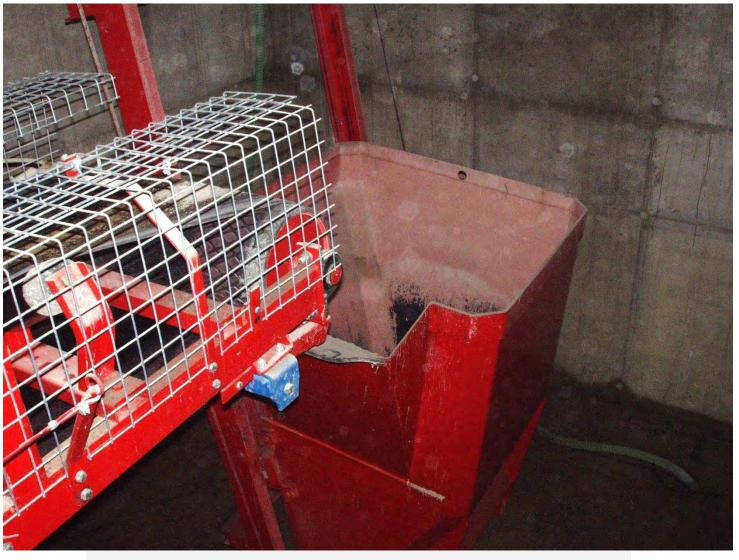
Aggregates batch unloaded inside skip in Germany
