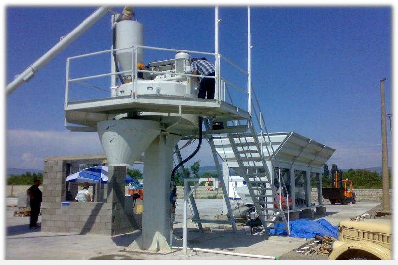
Assembling of compact Concrete Batching Plant manufactured by CM of small dimensions for a client in Tbilisi, Georgia
